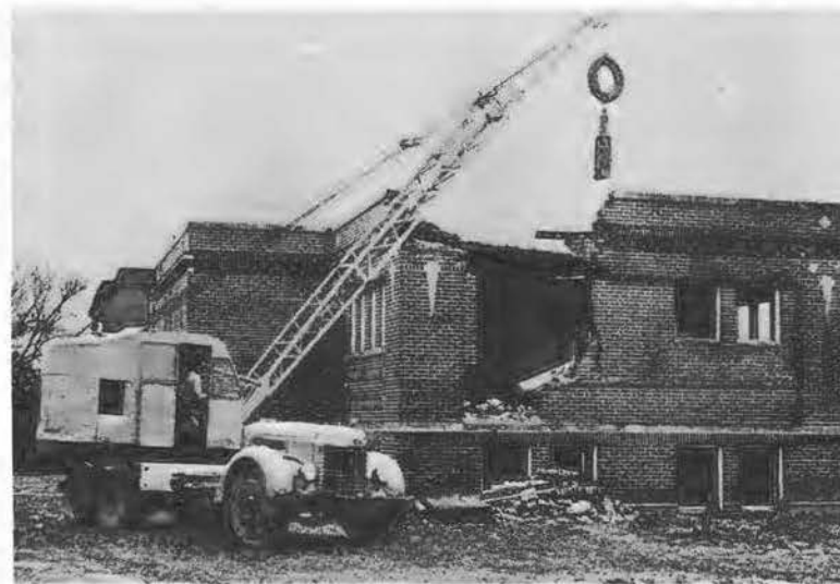
CLEARING GROUND for the Fine Arts Building.
