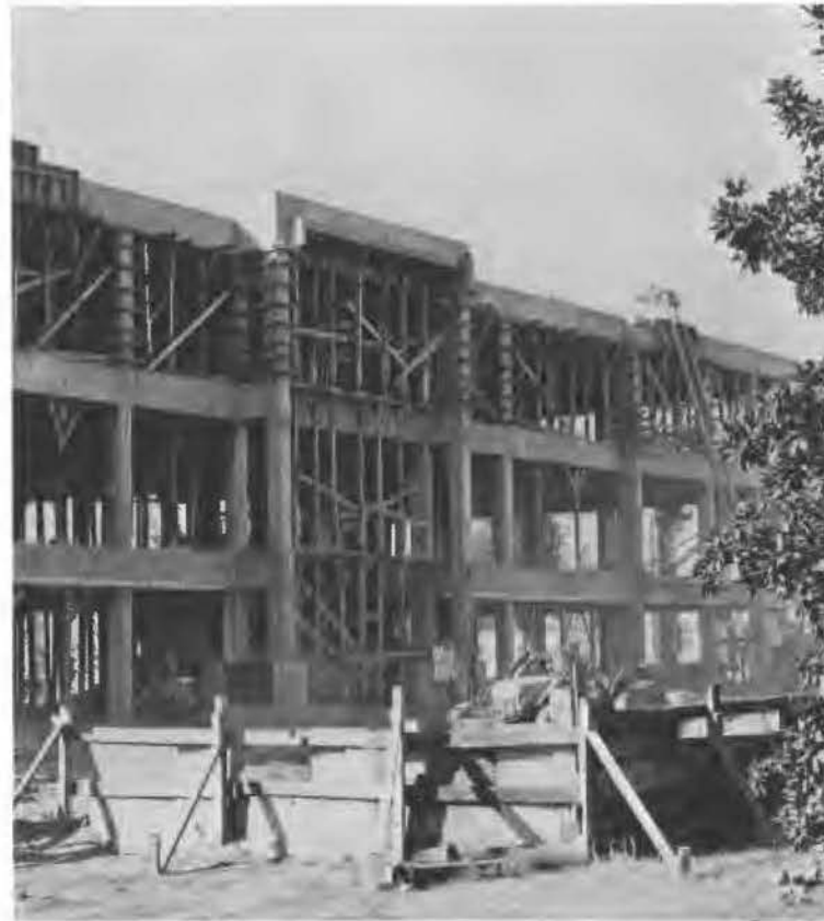
THE CLASSROOM building going up on campus.
